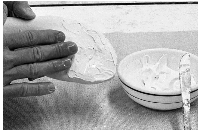
94 Shape and smooth the plaster.
